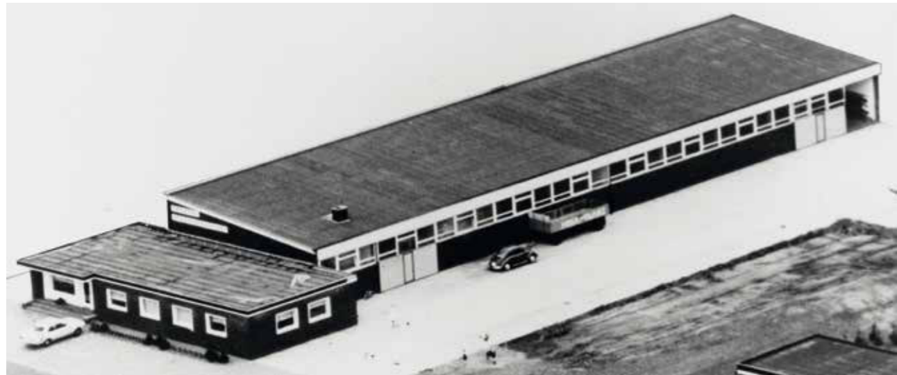
The first VEKAPLAST factory in Sendenhorst, 1969.
